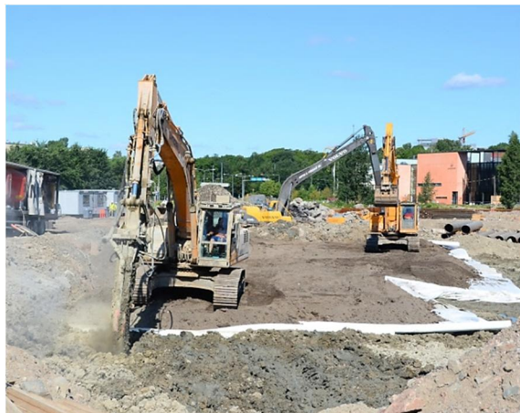
Figure 9. Arcada II. In the front left of the figure the binder is mixed with the abandoned soil with mass stabilisation machine. On the back right the compression embankment is being spread. (Arcada II; 14.7.2011)
