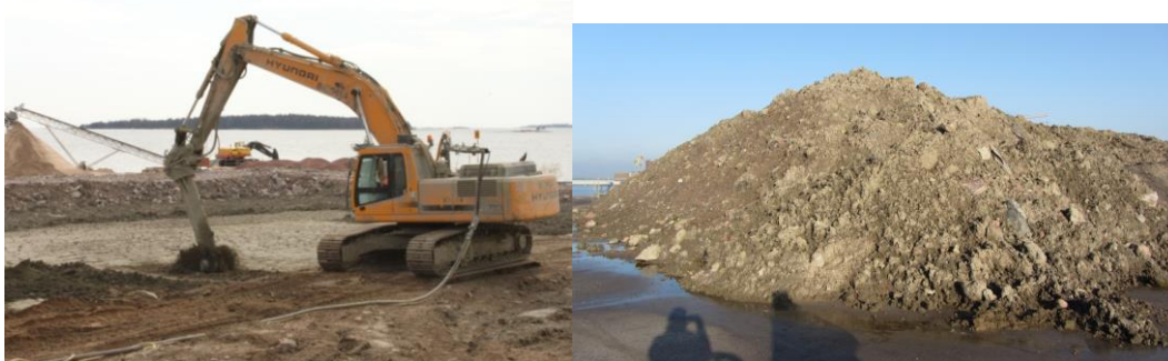
Figures 18-19. Jätkäsaari I/ Stabilisation in progress and stockpiled stabilised sediments waiting for transportation and further utilisation.
