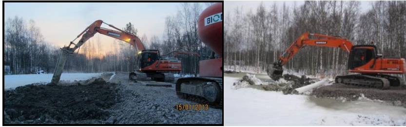
Figures 26-27. Stabilisation works in Dog Park carried out in winter time.
