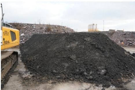
Figure 37. Test embankment – smaller noise barrier constructed with sediments stabilised with a crusher screener
