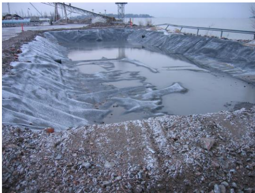
Figure 15. Stabilisation basins ready for filling with dredged sediments.
