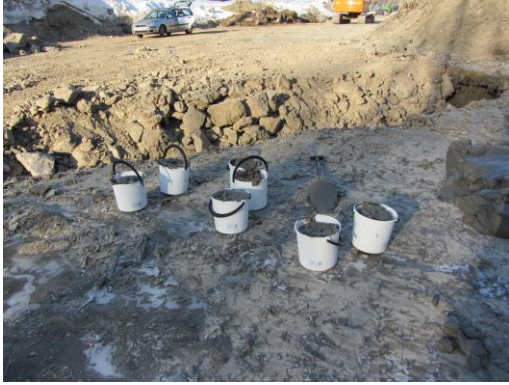
Figure 2: Samples collected from the place adjacent to the Dog Park that constituted a source of the additional surplus soils required for the fillings in this area. The redundant soil (very soft clay) came from mass replacement from a street construction behind the Dog Park.
