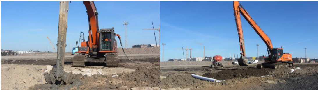
Figures 35-36. Jätkäsaari III: stabilisation work in progress. Geotextile is spread after stabilisation and the settlement embankment load placed on top.
