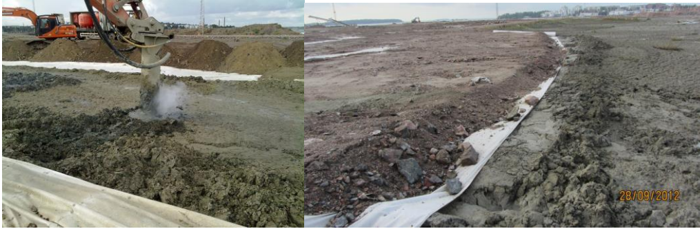
Figures 33-34. Jätkäsaari II - stabilisation in progress and sealing layer on top of the stabilised sediments.
