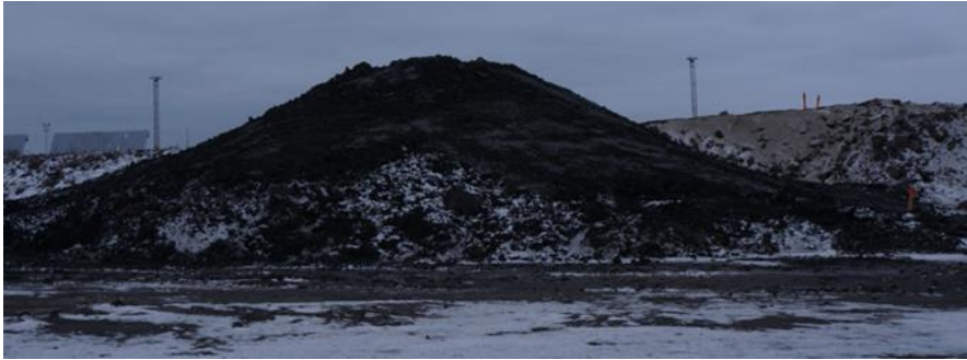
Figure 38. Larger test noise barrier constructed with mass stabilised sediments
