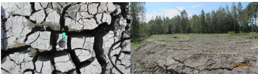
Figures 22-25. Surplus clays transported from other sites to the Dog Park as filling waiting for the start of stabilisation works.
