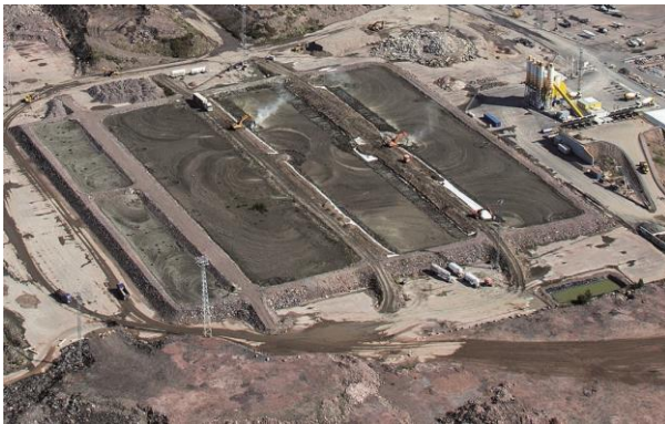
Figure 32. Aerial picture of the sedimentation basins. Stabilisation in progress in basins 1 and 2.
