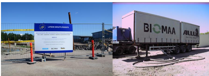
Figures 10-13 Stabilisation works in progress in Arcada 2 (Helsinki)
