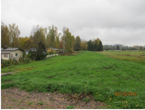
Figure 31. The new flood prevention dike was constructed with surplus clays originating from other construction sites in Vantaa in May-June 2012. The situation in October 2012.
