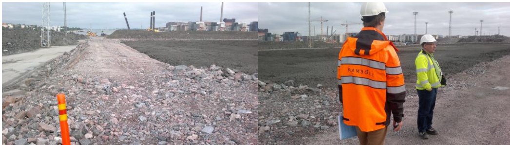
Figures 16-17. Stabilisation basins filled with dredged sediments.
