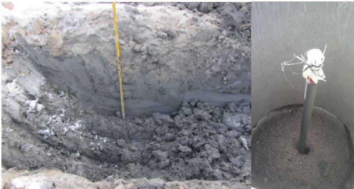
Figures 47-48. Jätkäsaari II - test pit. Settlement plates installed 9n May 2013.
