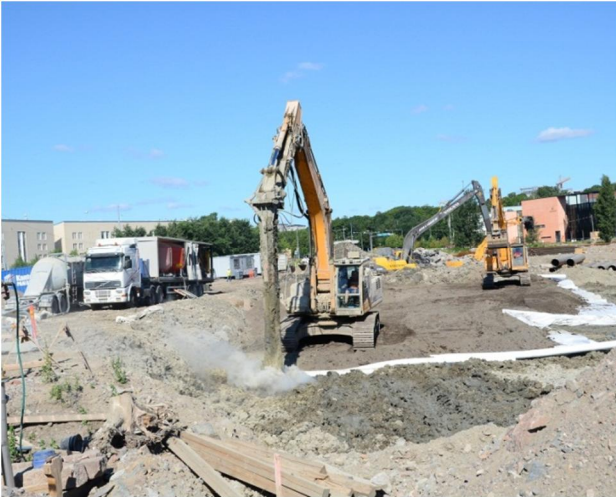
Figure 11.9 Mass stabilisation in progress
