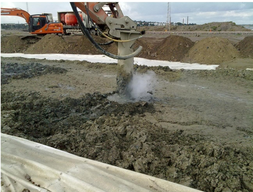
Picture 12.18 Stabilisation in progress
