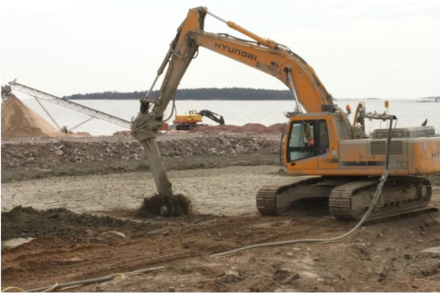
Figure 12.7-12.8 Jätkäsaari I – stabilisation works in progress
