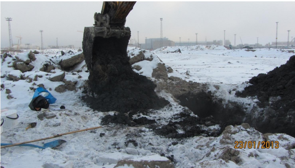
Picture 12.21 Test pit digging
