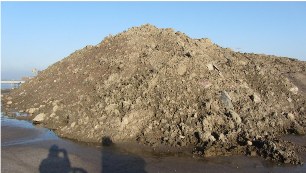
Figure 12.9 Mass stabilised sediments stockpiled and waiting for reuse in 2012
