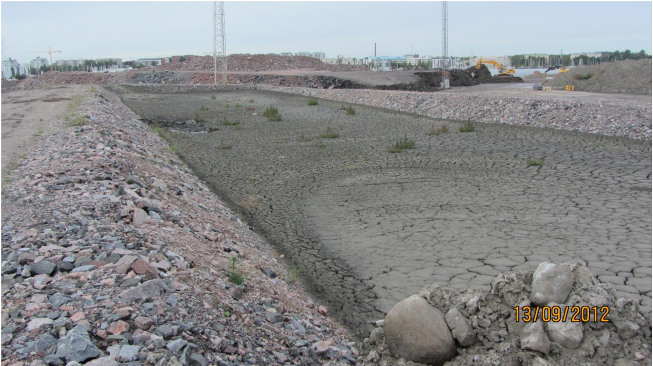
Picture 12.11 Sediments waiting for stabilisation in a basin.
