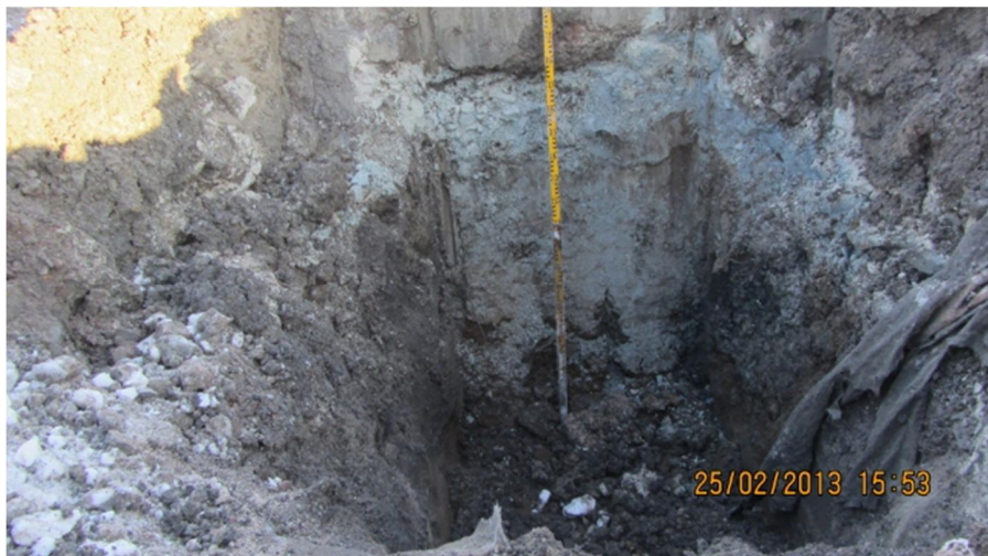
Figure 7.5 Excavating test pits; documentation and depth profiling
