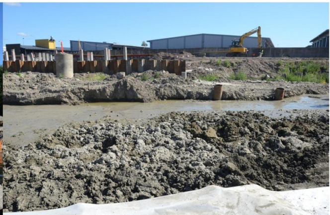
Figure 11.12 Stabilisation basin – satbilised clay in front, clay waiting for stabilisation at the back
