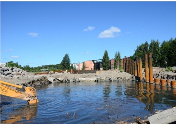
Figure 11.11 Removal of original filling
