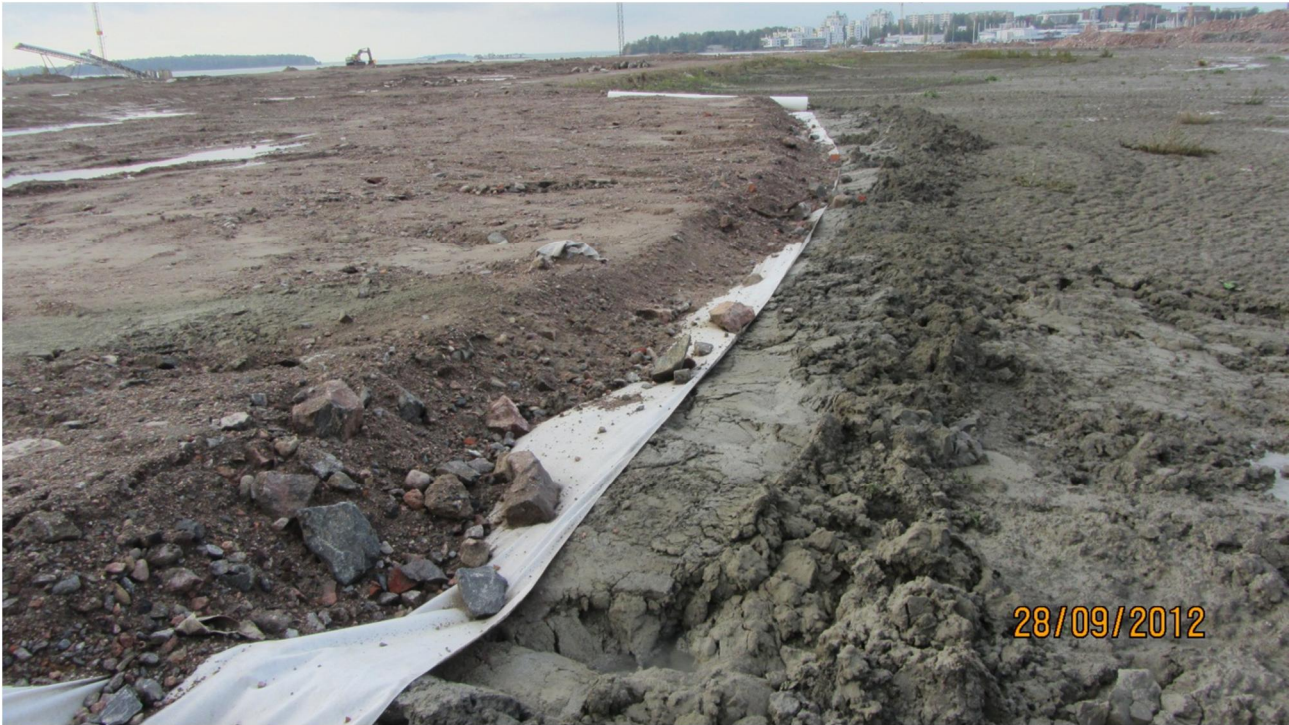
Picture 12.19 Sealing layer on top of the stabilised sediments
