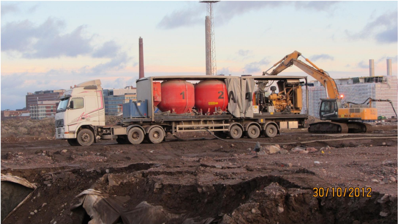
Picture 12. 17 Pressure feeders
