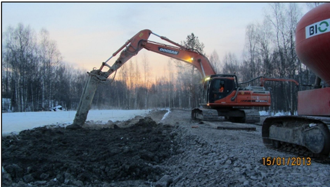
Figure 5.2 Mass stabilisation work carried out in winter conditions in Espoo, Finland (15.1.2013)
