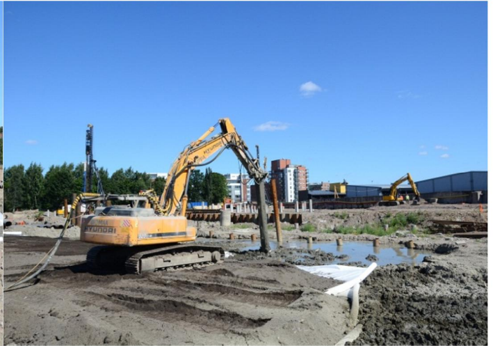
Figure 11.10 Piling works in progress
