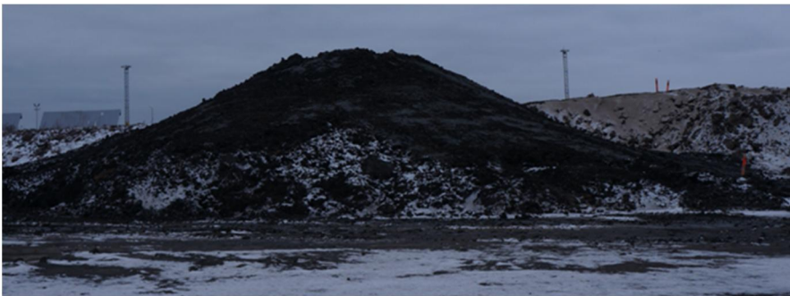
Picture 12.27 Larger test noise barrier constructed with mass stabilised sediments (2015)
