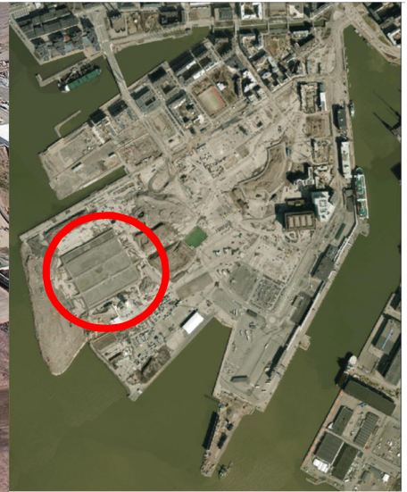
Fig. 12.3 Mass stabilisation basins in the West harbor.
