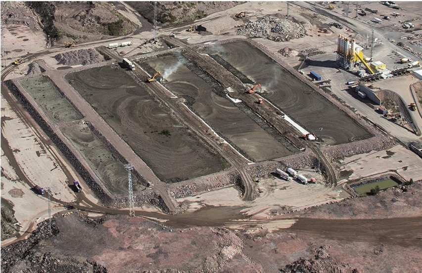
Fig. 12.2 Mass stabilisation phase II, autumn 2012. Basin number 1 right (near ready-mixed concrete plant) and no. 2...4 to left.
