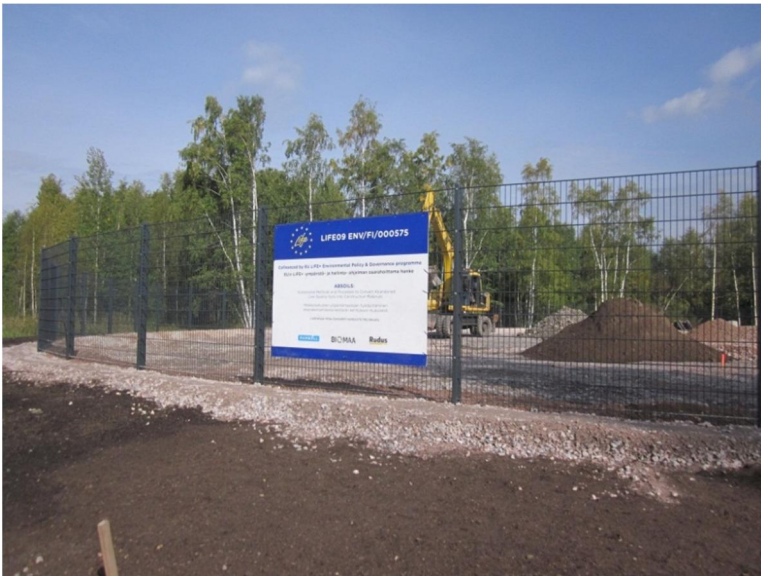
Figure 10.1 Perkkaa Dog Park under construction in September 2013.
