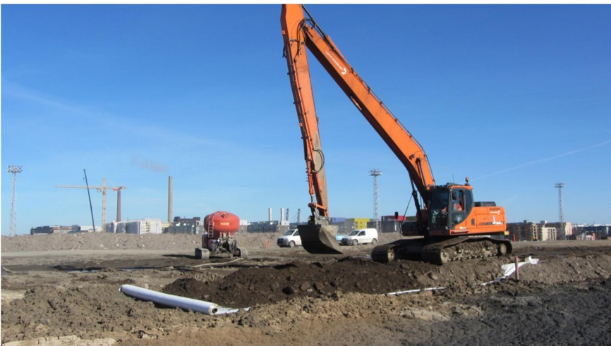
Picture 12.24 Jätkäsaari III : geotextile is spread after stabilisation and the settlement embankment load is placed on top
