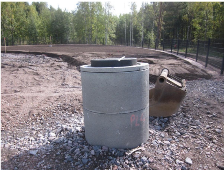
Figure 10.2 Concrete wells for lysimeters and settlements plates.
