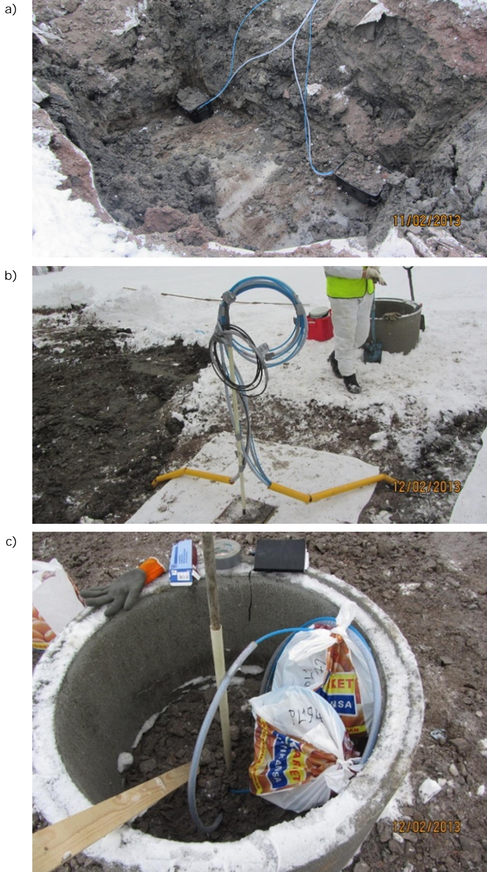
Figure 8.13 Lysimeter installation details a) installed lysimeters before filling b) & c) technical details of lysimeter tubing protection and covering in concrete wells
