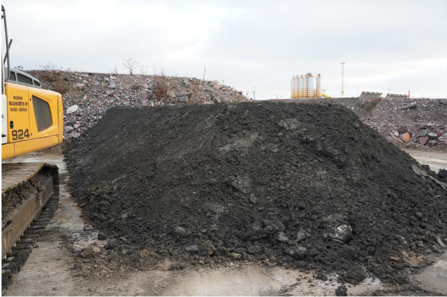
Picture 12.26 Test embankment – smaller noise barrier constructed with sediments stabilised with a crusher screener (2015)
