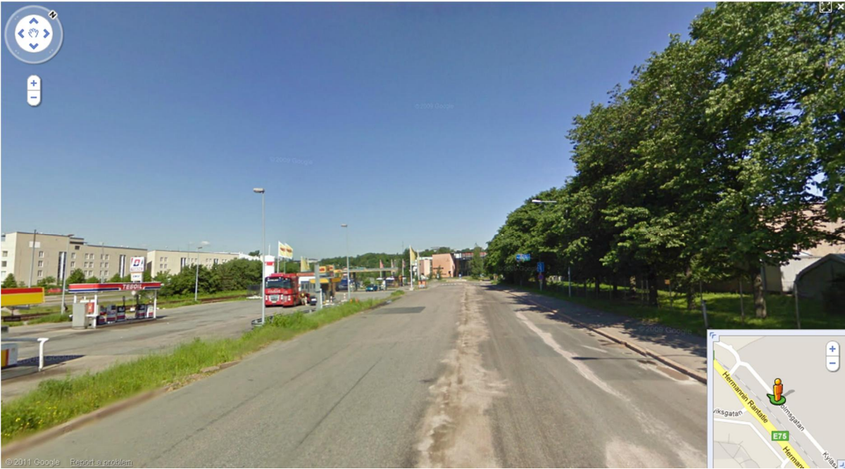
Figure 11.2 Arcada II before construction. (Google maps)
