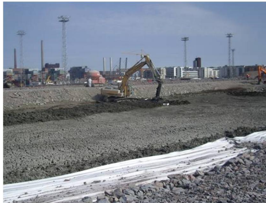
Fig 16. Stabilisation work in basin 2, 2011 (in the front right corner - loading embankment and geotextile; at the back - stabilisation machine running)
