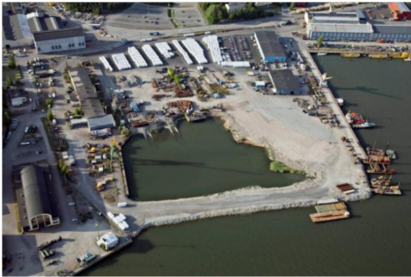
Fig 8. Stabilisation and filling basin of the Pansio port
