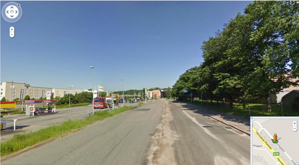
Figure 1. Arcada 2 before construction. (Google maps)
