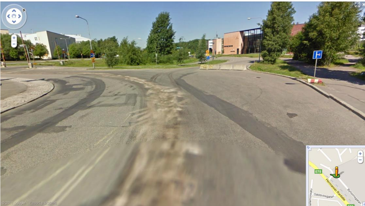
Figure 2. The last part of the road blocked for entrance and the road has been pached with asphalt. (Google maps)
