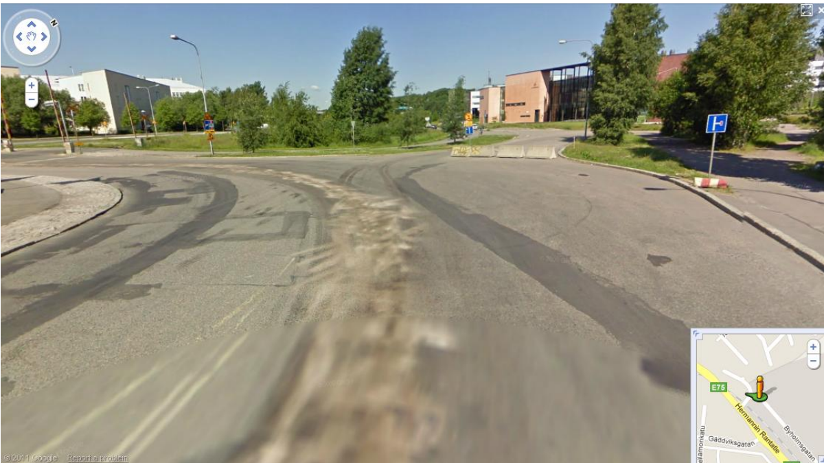
Figure 2. The last part of the road blocked for entrance and the road has been pached with asphalt. (Google maps)
