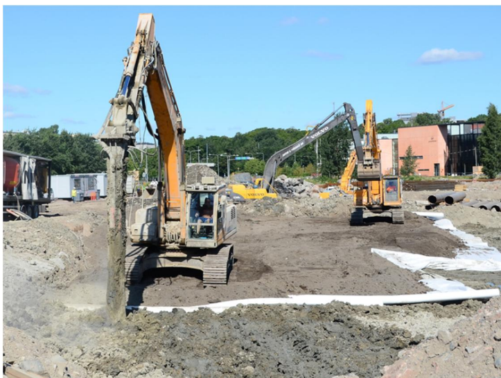
Figure 4.2 In situ mass stabilization at the Arcada2 pilot site (2011).
