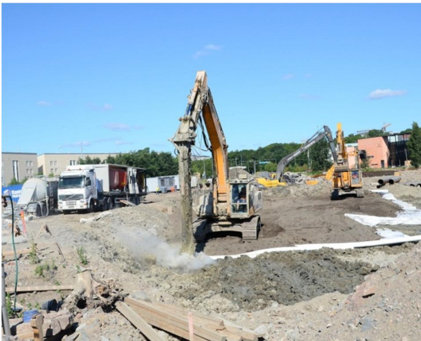
Figure 5.6 Mass stabilization in progress
