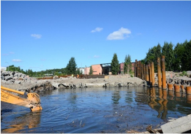
Figure 5.8 Removal of original filling
