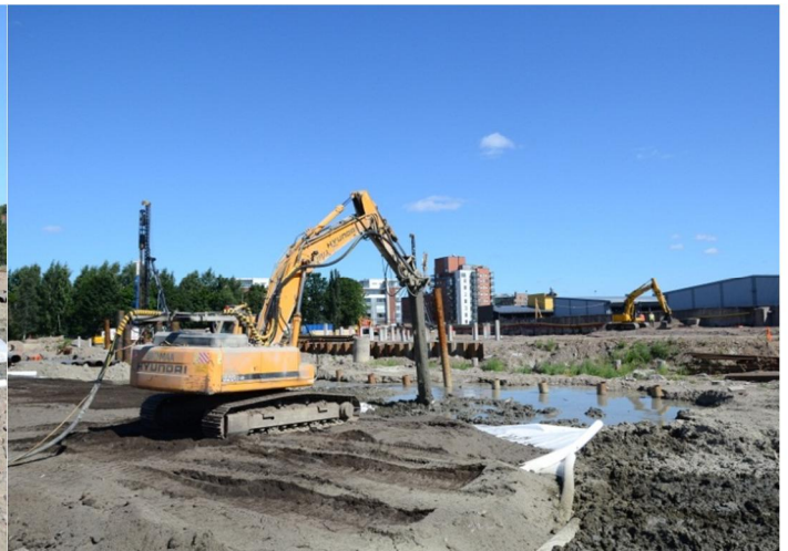
Figure 5.7 Piling works in progress
