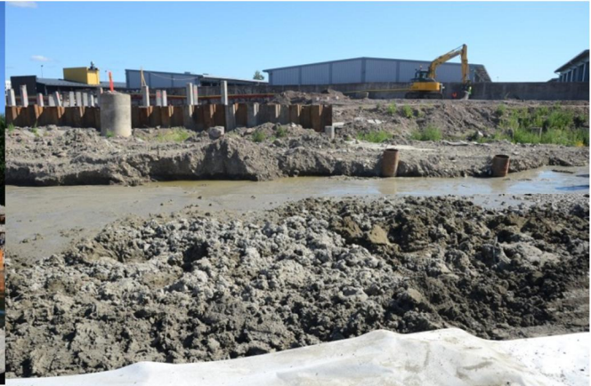
Figure 5.9 Stabilization basin – stabilized clay in front, clay waiting for stabilization at the back
