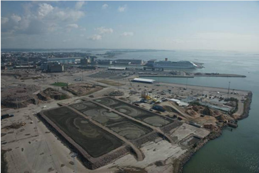
Figure 4.5 Mass stabilization basins of the Jätkäsaari I pilot (2011)
