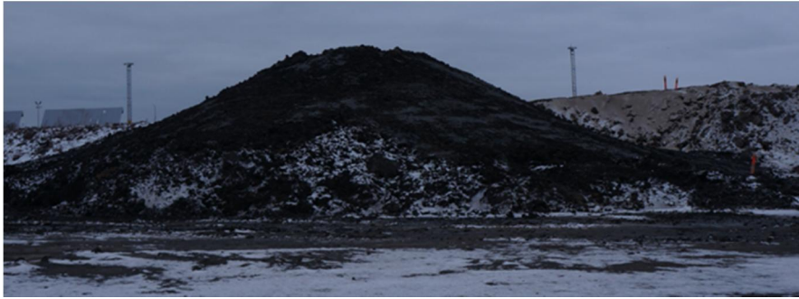
Figure 5.4 Test noise barrier constructed with mass stabilized sediments– Jätkäsaari III pilot site (2015)
