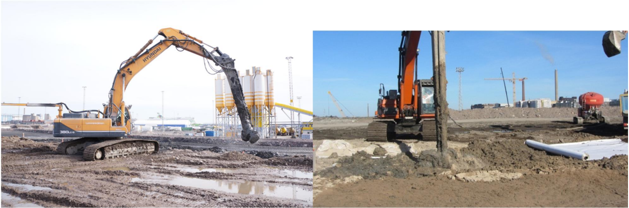
Figure 1.2 – 1.3 Mass stabilization process at the Absoils pilot site: Jätkäsaari, Helsinki
