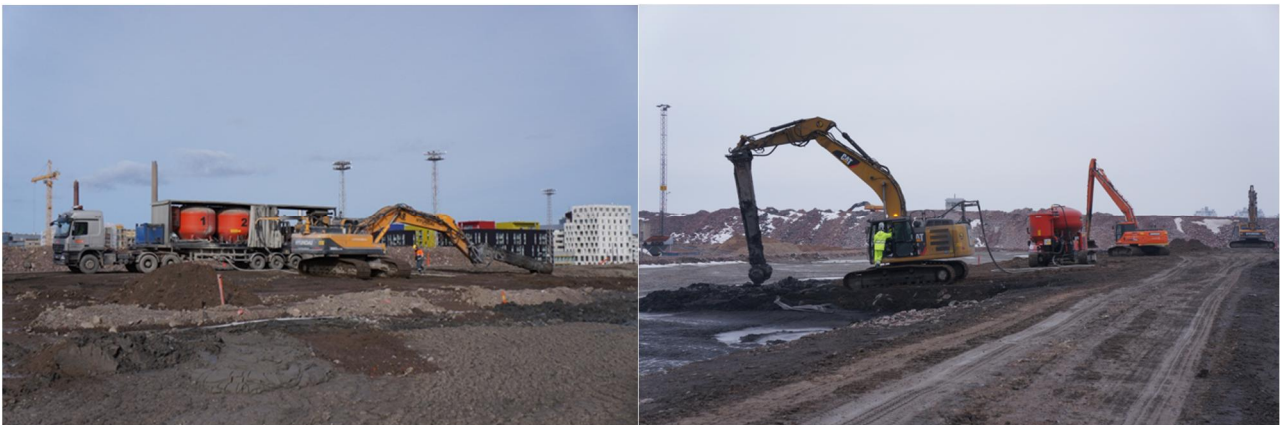
Figure 2.1 – 2.2 Mass stabilization basic equipment with the mixing unit attached to the excavator and connected to the pressure feeder.
