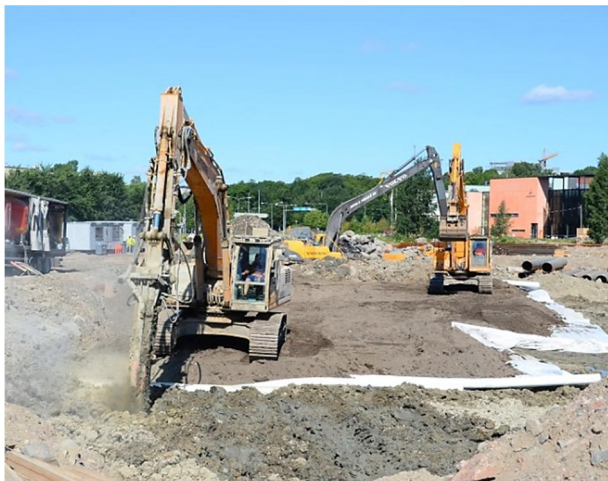
Fig. Arcada II. Mass stabilisation on-going.
