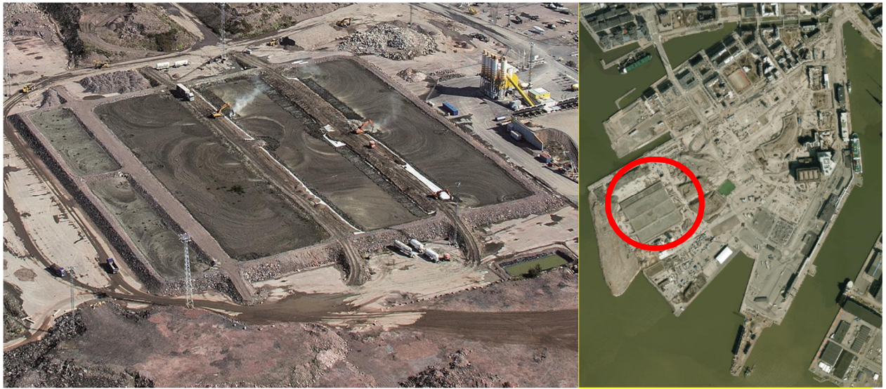
Fig. Mass stabilisation phase II, autumn 2012. Basin number 1 right (near ready-mixed concrete plant) and no. 2...4 to left.
