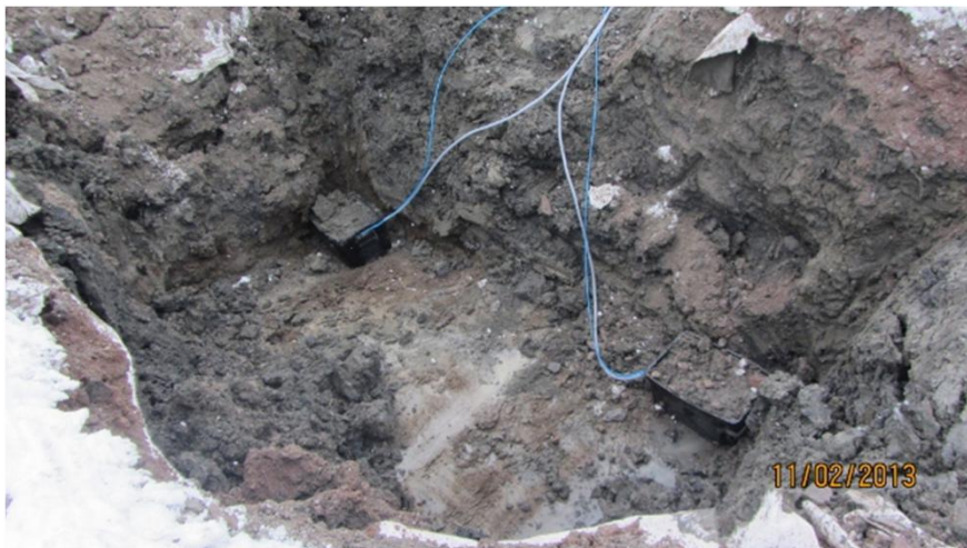
Installing lysimeters 11.2.2013
