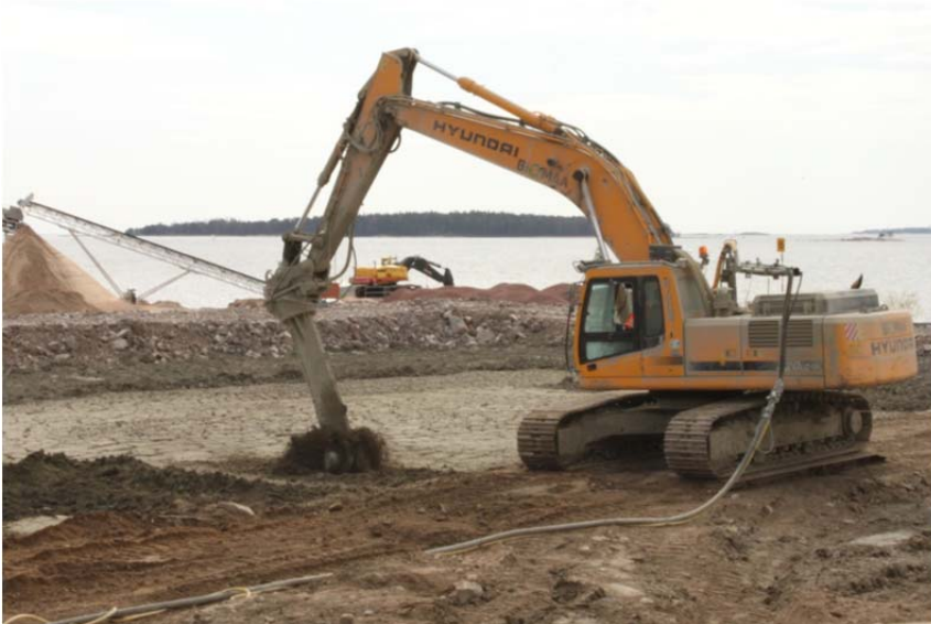
Figure 2. Stabilisation in progress in Jätkäsaari I pilot application.
