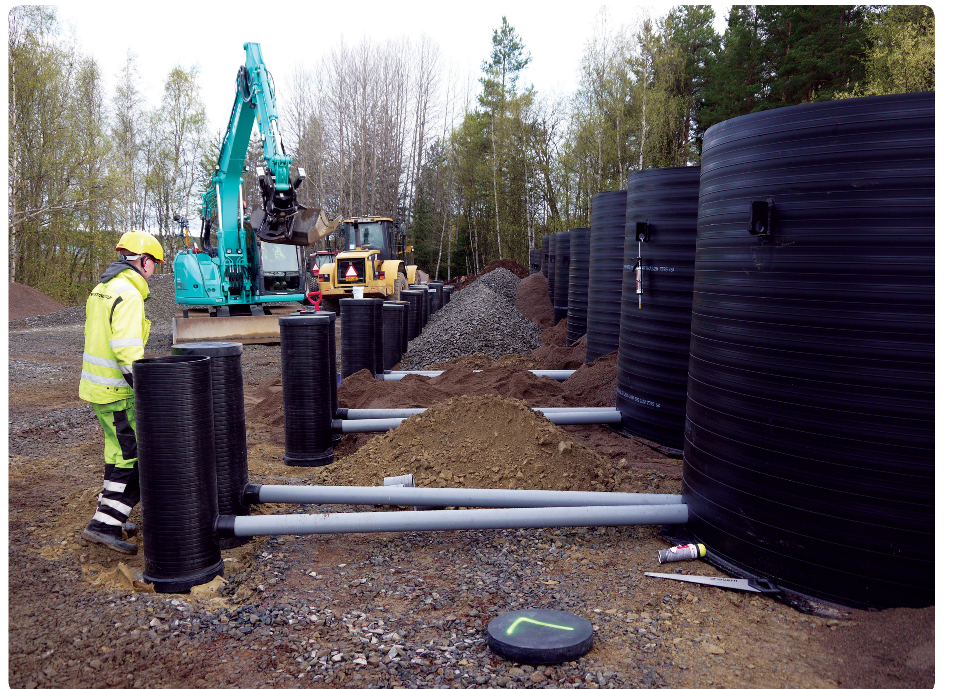
Figure 2. Field tests in Pyhäsalmi Mine. 10 lysimeters were built in 2016.
