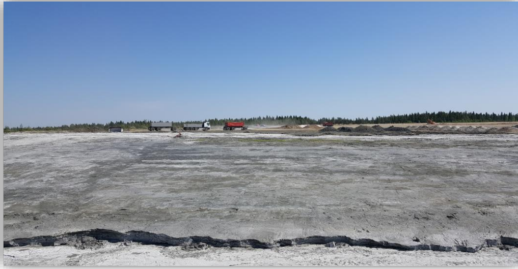
Levelled enrichment sand waiting to be covered
