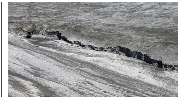
Levelled enrichment sand before covering it with fibre clay
