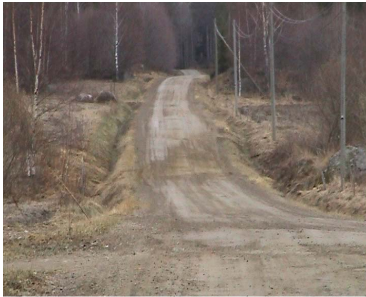
Frost damage of a gravel road (Luopioinen 2002)
