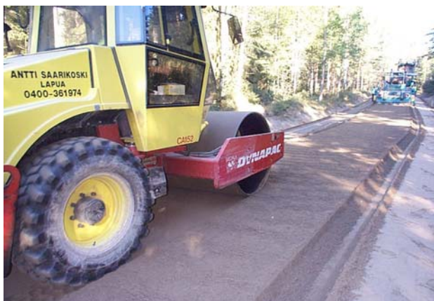
Spreading of the binder admixture
