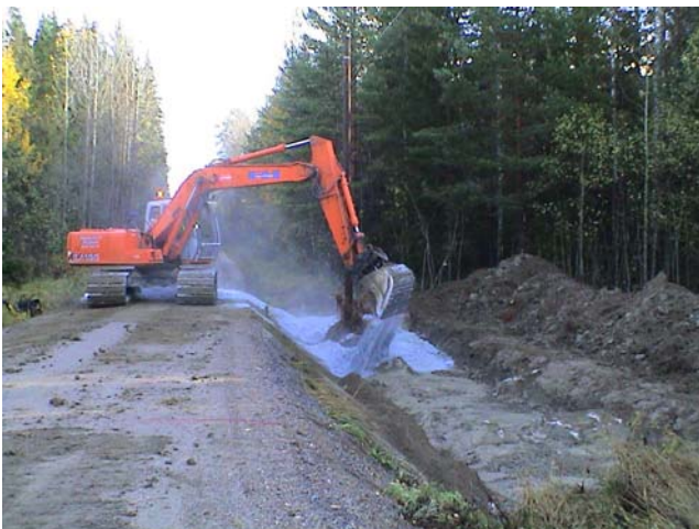
Spreading of fibre-ash on the planed road surface
