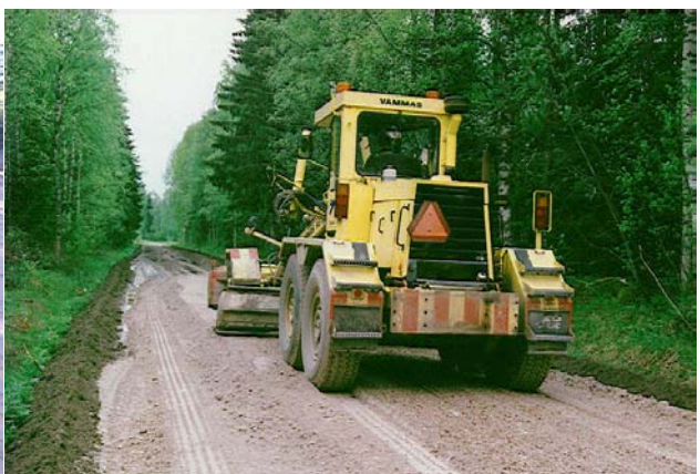
Stabilisation with a milling cutter
