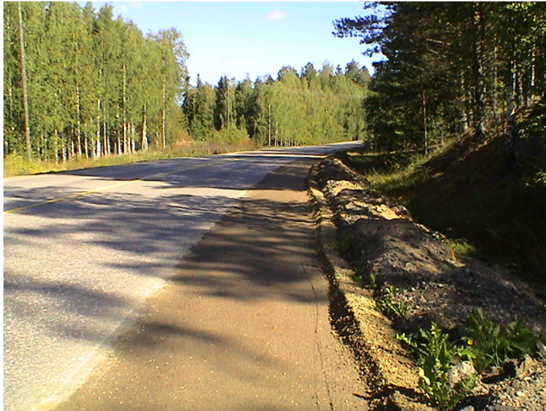
Figure 11: The safety lane before finishing. Luopioinen, early autumn 2003.
