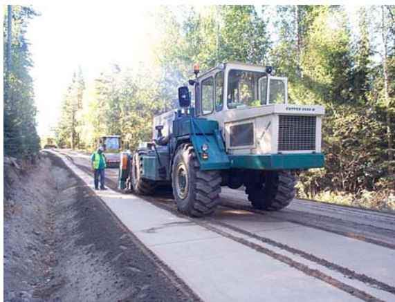
Figure 3: Stabilisation in progress: a milling machine at work
