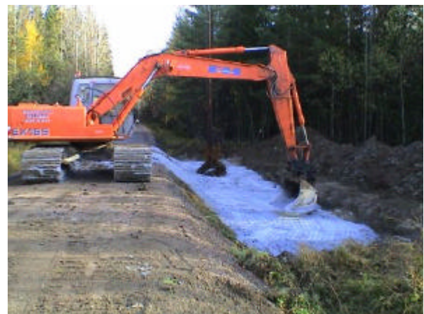
Figure 6: Compaction of the fibreclay for the groundwater protection structure's sealing course.
