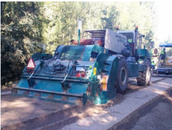
Figure 4: Stabilisation process in 2002. In the front the milling cutter.
