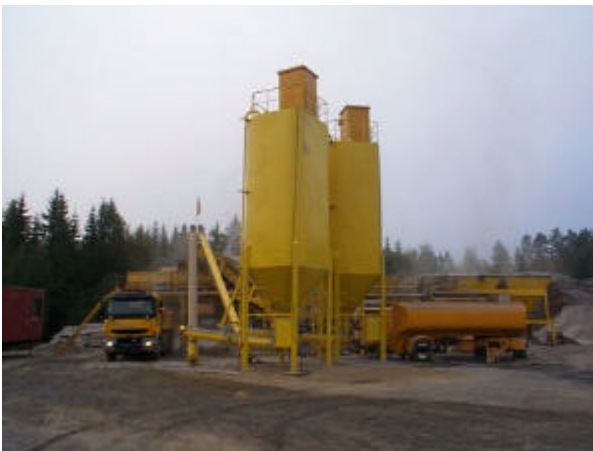
Figure 3: Mixing station for binder admixtures in 2002.
