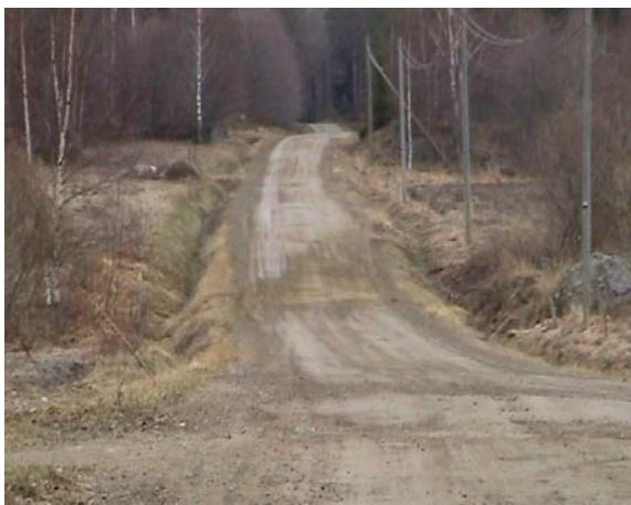
Figure 7: The village road in the spring 2003, before renovation. Pilot 2003
