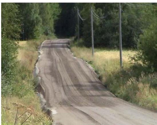
Figure 8: The village road in the autumn 2003, after the renovation operations. Pilot 2003
