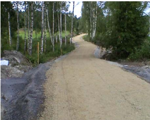
Figure 6: A section of light-traffic lane before finishing. Pilot 2003
