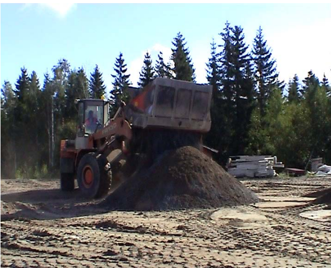
Figure 2: Mixing shovel at work to mix crushed aggregate with filterwaste. Pilot 2003
