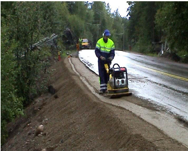
Figure 5: Compaction on the safety lane. Pilot 2003
