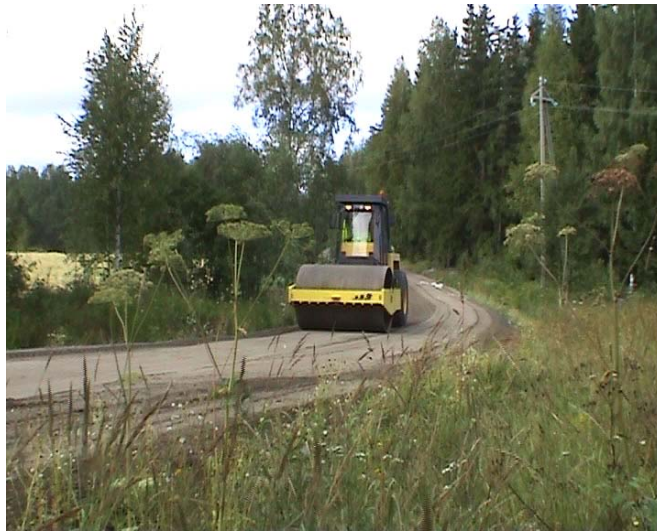
Figure 3: Compaction of the fibre-ash course covered with crushed aggregates. Luopioinen 2003.
