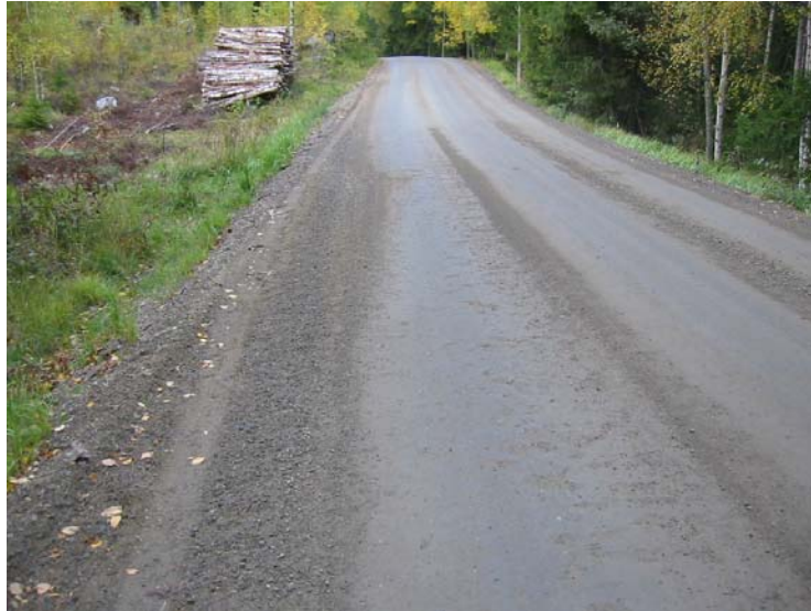
Figure 5: The thickness of the covering course varies significantly in the autumn 2003, one year after the construction of Pilot 2002. Ramboll Finland Oy 2003.
