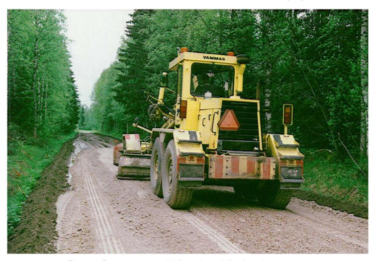
Figure 6: Covering course with filtercake-stabilised crushed stone
