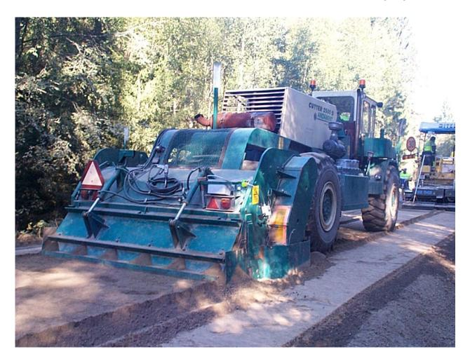
Figure 4: Stabilisation with a milling cutter
