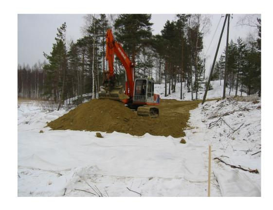
Figure 16: One of the lanes was constructed on soft (peat) soil; therefore the first tasks were to preload the site some months before the construction
