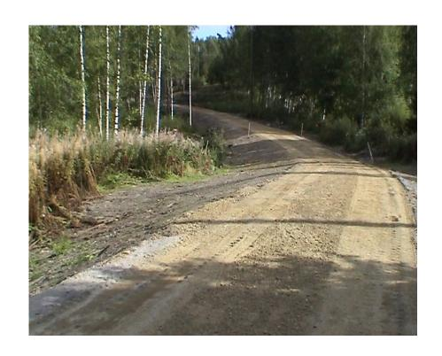
Figure 18: The light-traffic lane (and the fibre-ash course) covered with crushed aggregate mixed with filter cake
