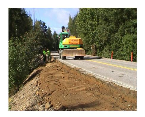
Figure 21: The road sides have been opened and planed for the geonet and fibre-ash course
