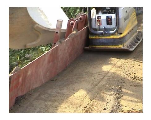
Figure 23: The fibre-ash course is covered thinly with crushed aggregate, and the safety lane can be compacted
