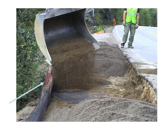
Figure 22: Fibre-ash is being spread over the geonet. Note the metal plate support for a steep road edge.
