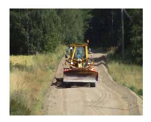
Figure 9: Planing and forming of supporting edges for the fibreash course
