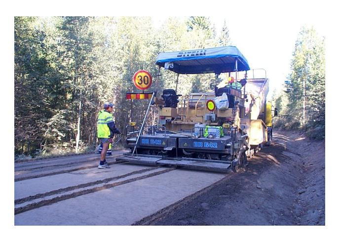
Figure 3: Spreading of binder admixtures
