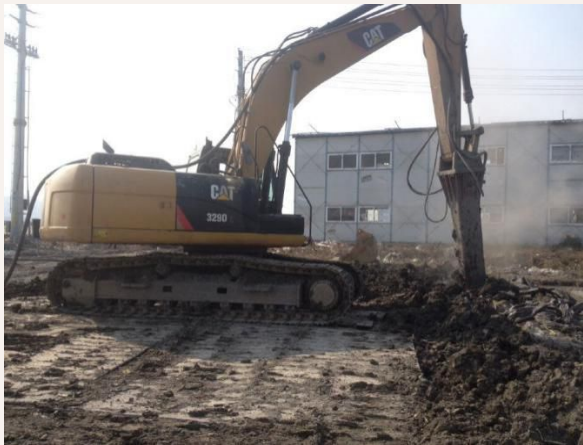
Precompress treated area
