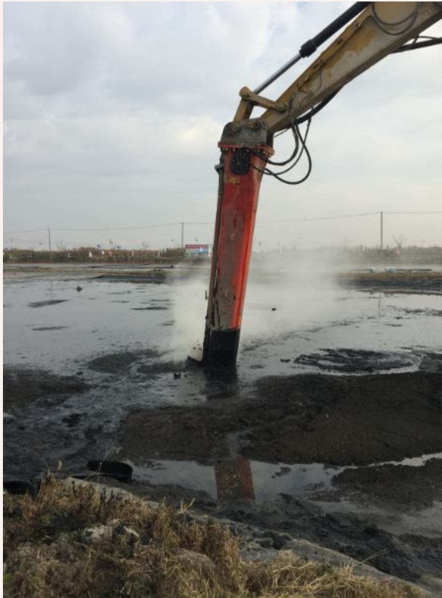
Contaminated soil (from sewage plant) treatment
