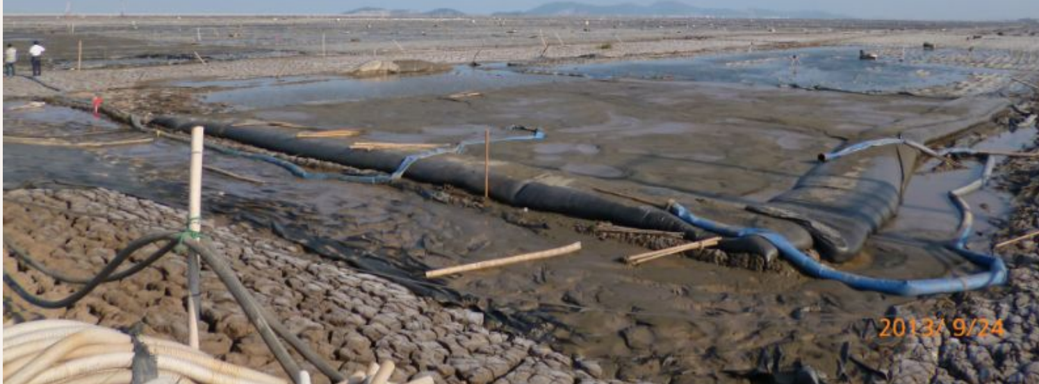
Reclamation area treated with Vacuum preloading
