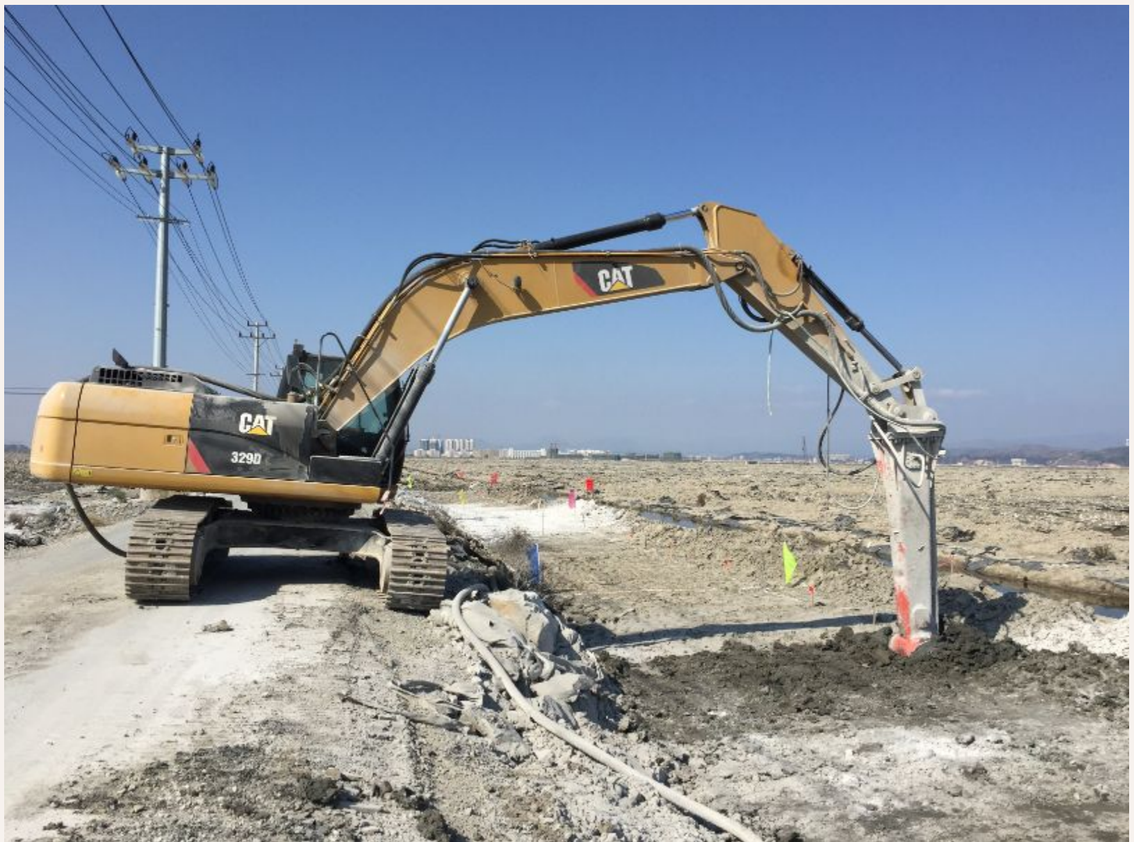
Mass stabilisation for hydraulic filled dredge (Wenzhou, China)
