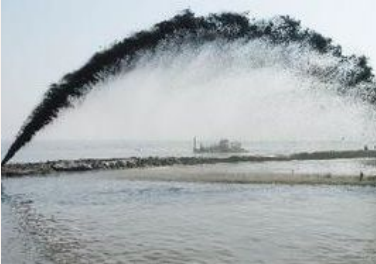
Hydraulic filling for ocean reclamation
