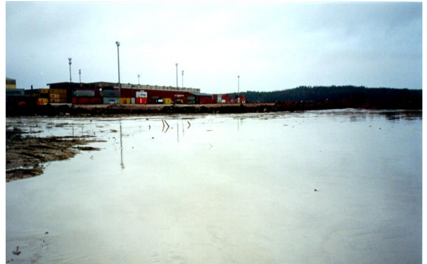
Mass stabilisation of dredged sediments at Hamina harbour 1996
