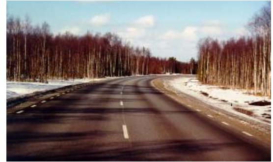
Road in use
