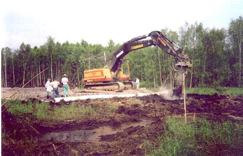
Mass stabilisation at Veittostensuo 1993
