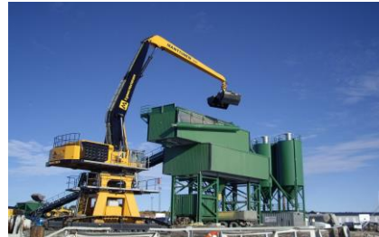
Process stabilisation, mass stabilisation in barge
