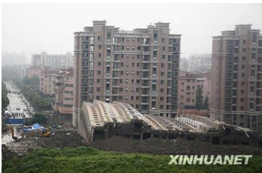
pile failure
