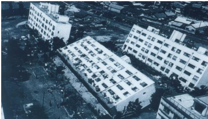
Liquefaction in 1964 earthquake
