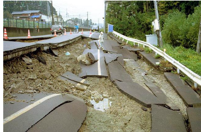
slope failure in 2007 earthquake
