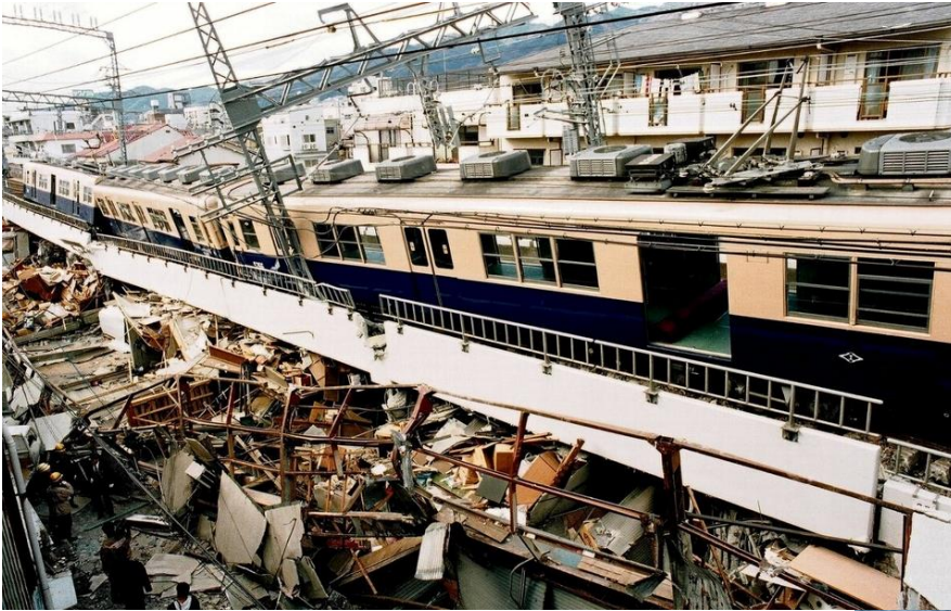
Earthquake attack in 1995 earthquake
