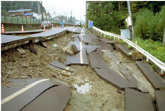
slope failure by earthquake
