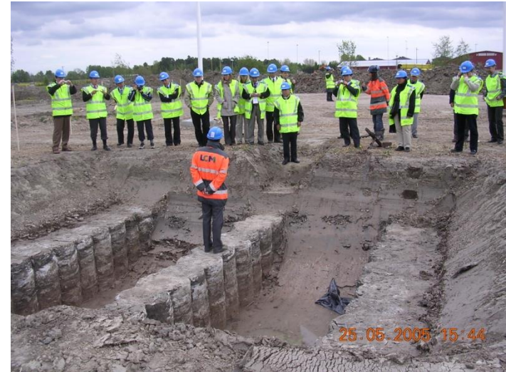
Exposed DDM columns for permanent slope stability in Uppsala – Sweden (2005)
