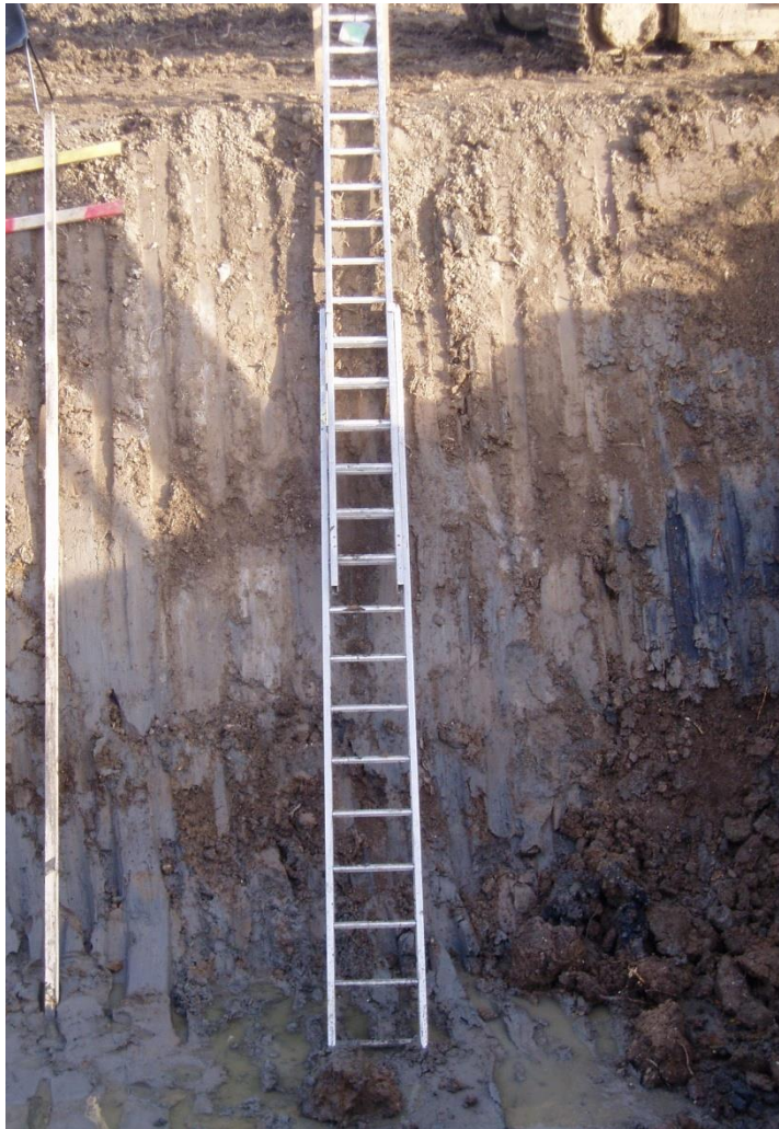
Temporary excavation pit Clay – UK (2005)
