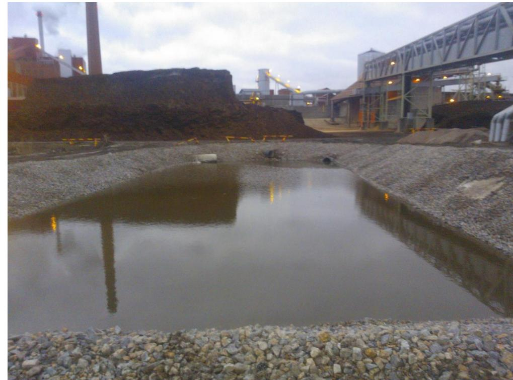
Water pools made to basin B, mass stabilised kaolin clay
