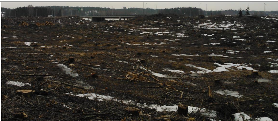
Situation before mass stabilization at project area
