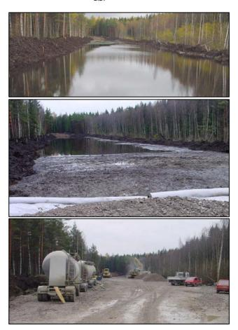
First mass stabilizations in Kivikonlaita – effect of stabilization
