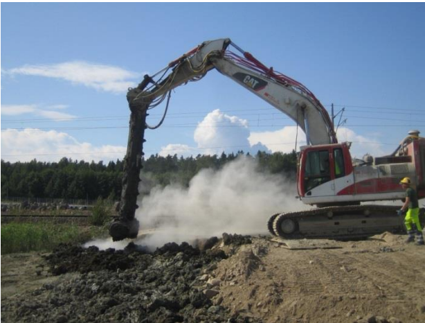
Mass and column stabilization in Kotolahti Railway yard in 2009
