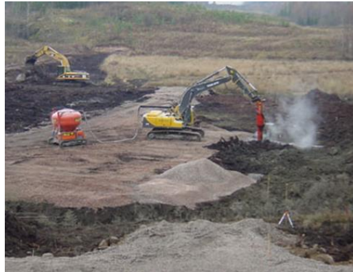
Mass stabilization ongoing at summer and winter conditions
