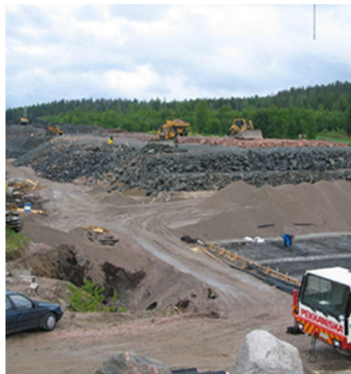
Construction of the railway base on top of the mass stabilized and piled subsoil (left) and ready track (right)
