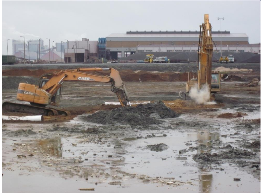
Ongoing mass stabilization
