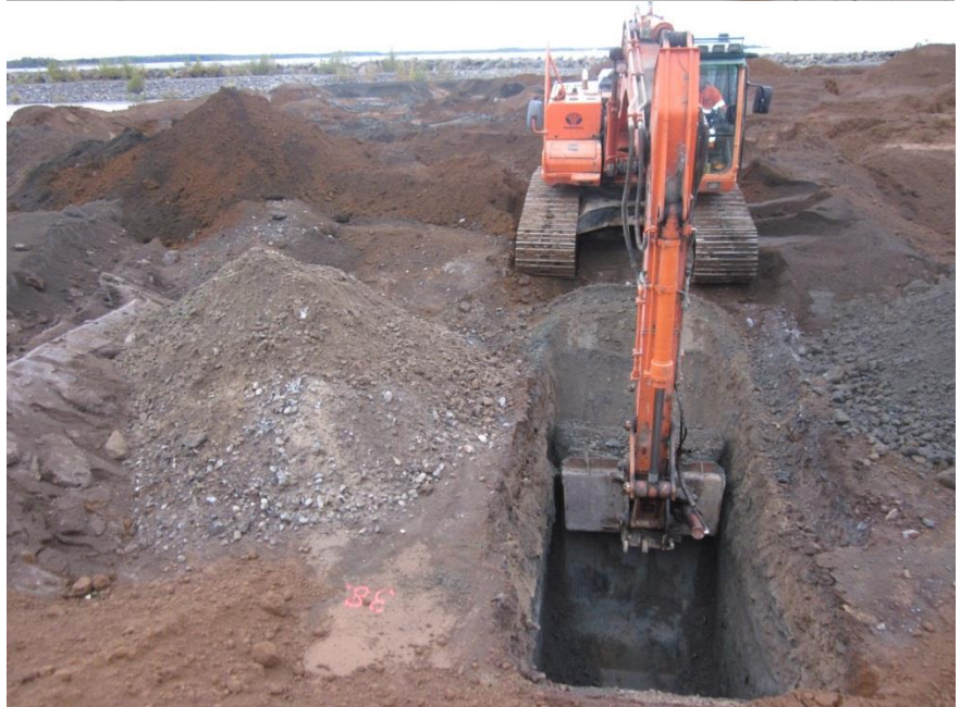
Test pit for technical quality control
