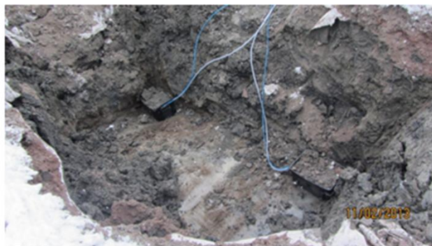
Installing lysimeters 11.2.2013
