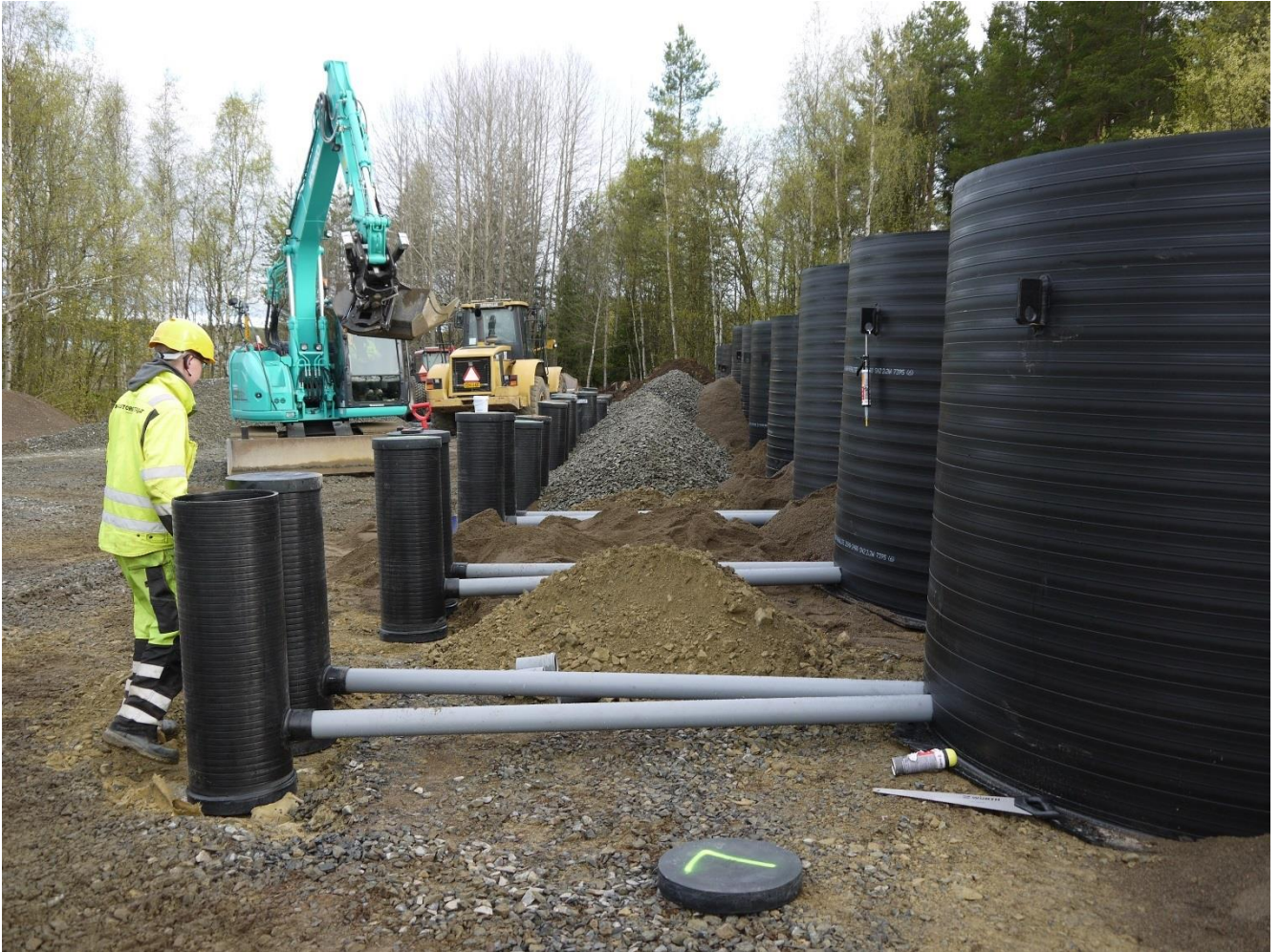
Figure 3. Field tests in Pyhäsalmi Mine. 10 lysimeters were built in 2016.
