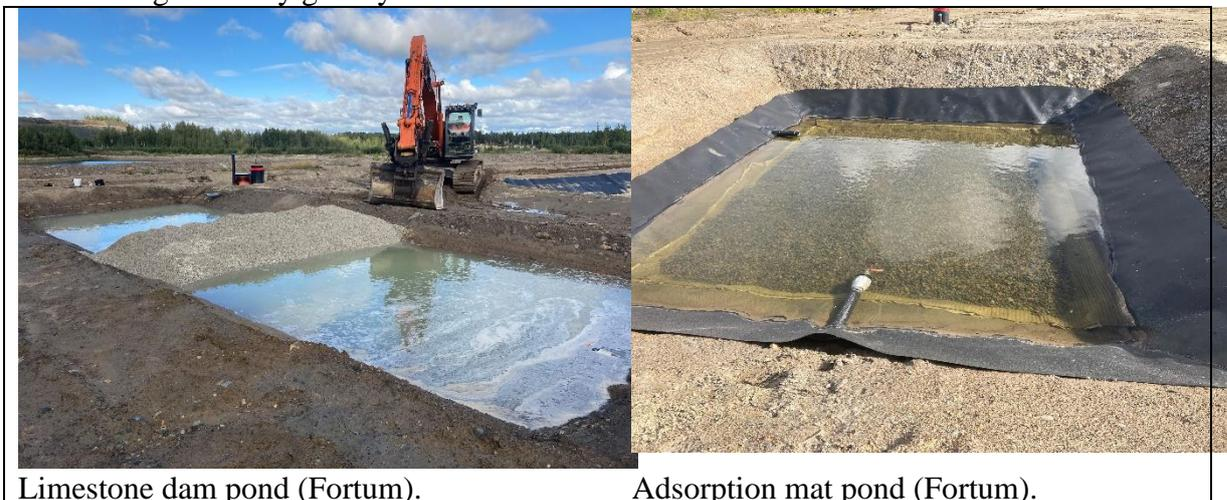
Figure 12. Reactive structure pilots 2021.
