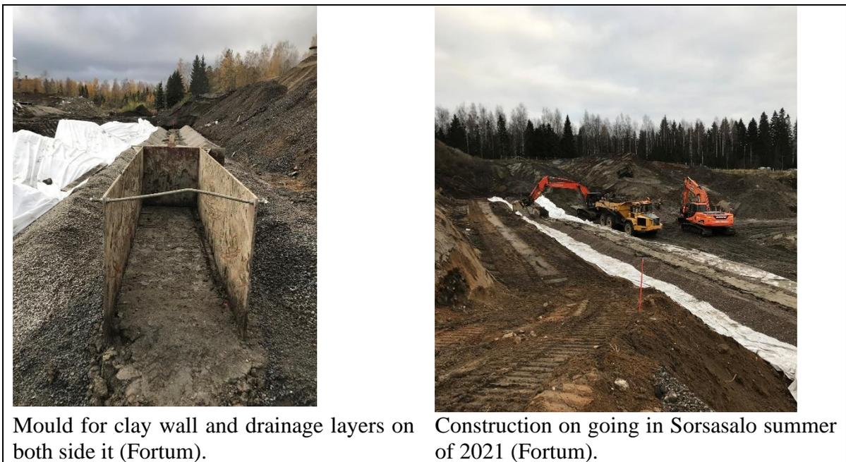
Figure 11. Pilot of vertical sealing layer in Sorsasalo.
