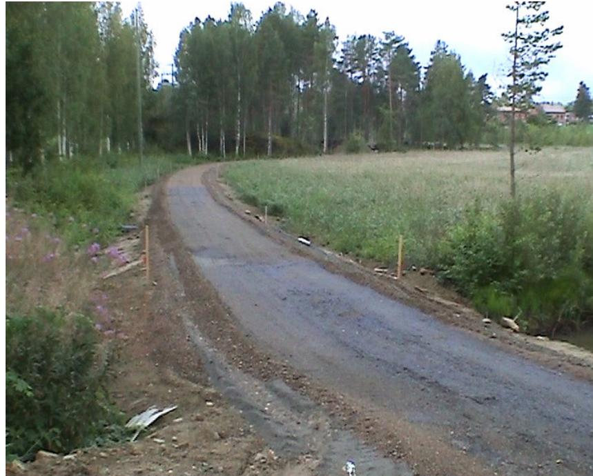
Figure 17: The light-traffic lane with edge supports and the fibre-ash course after compaction
