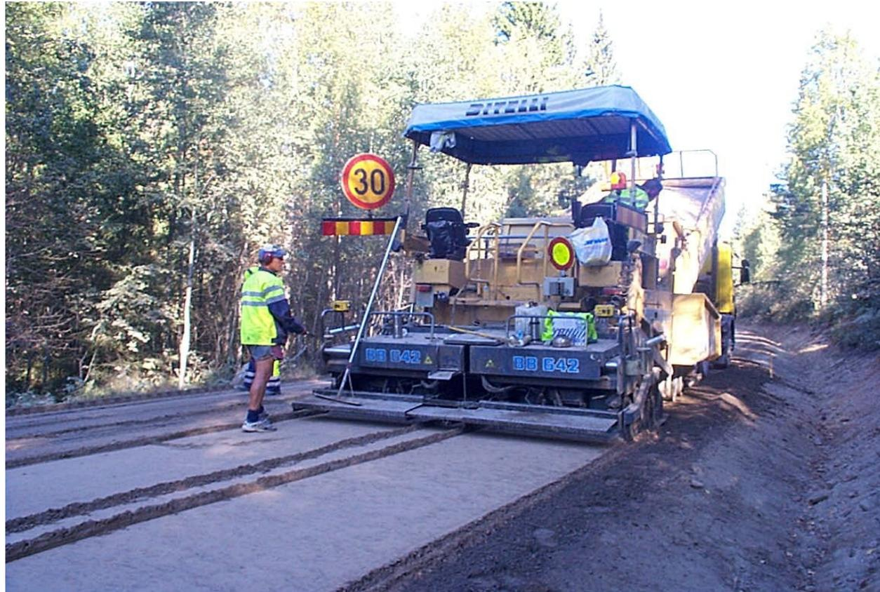
Figure 3: Spreading of binder admixtures
