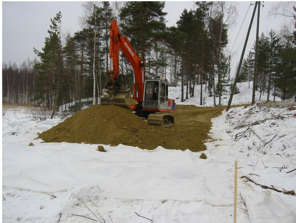
Figure 16: One of the lanes was constructed on soft (peat) soil; therefore the first tasks were to preload the site some months before the construction
