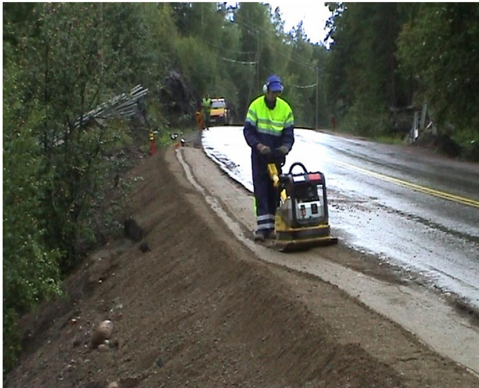
Figure 24: Finally the safety lane is covered with filtercake-stabilised crushed aggregate and compacted for the finish. The final touch will be given with separating marks in the summer 2004
