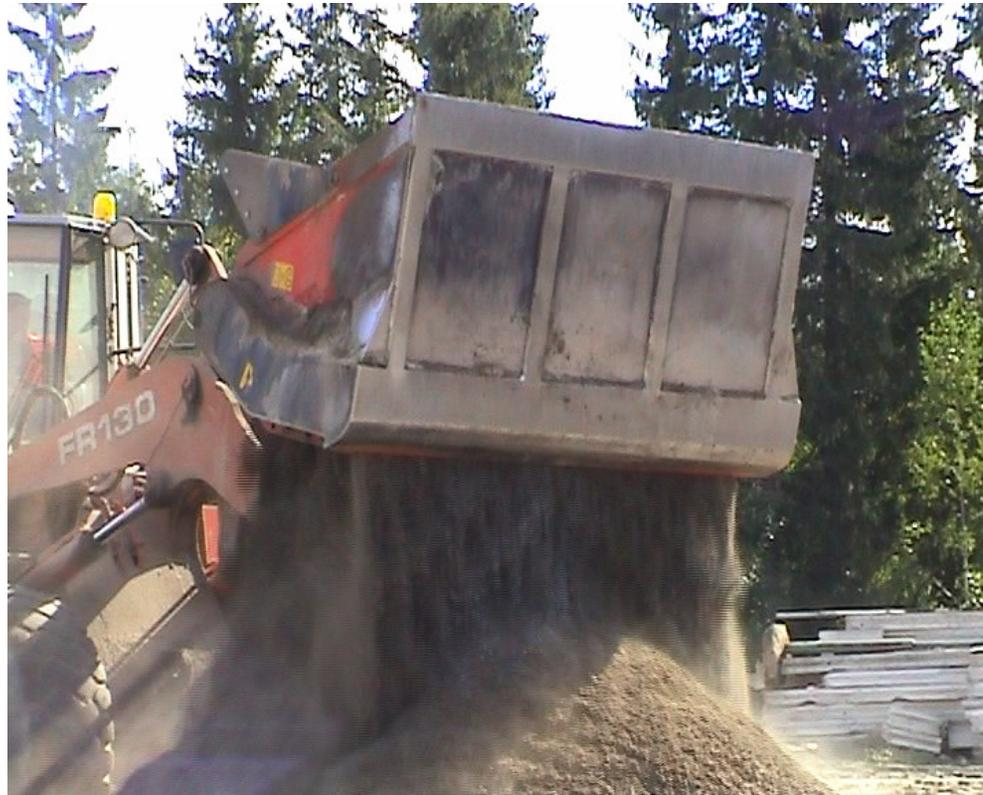
Figure 20: For smaller quantities the scoop mixing is adequate
