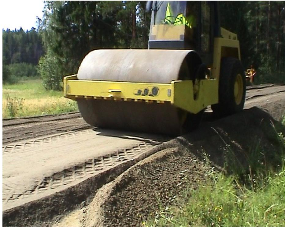
Figure 11: The renovated section is covered with a filtercake-crushed aggregate mixture, and compacted
