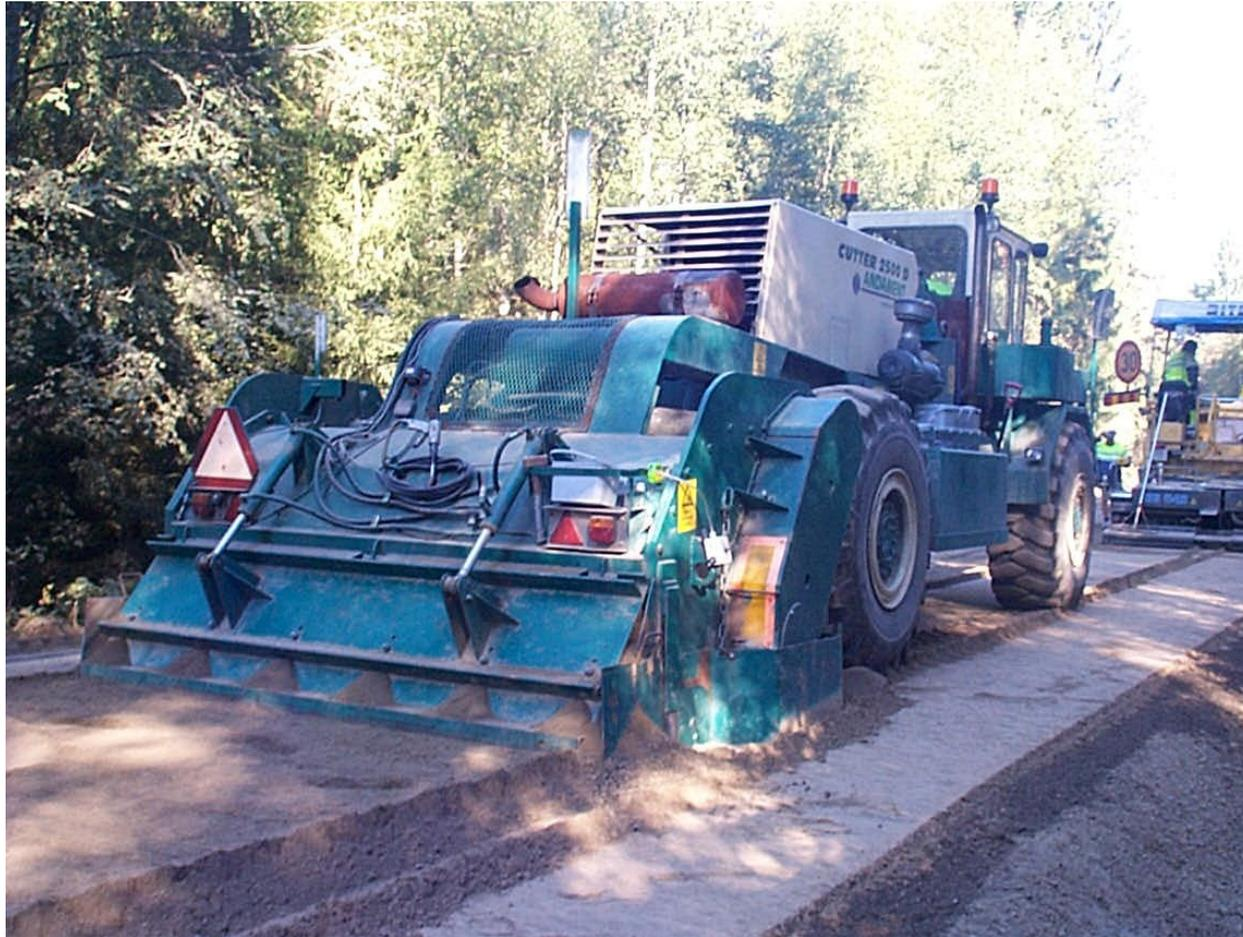
Figure 4: Stabilisation with a milling cutter
