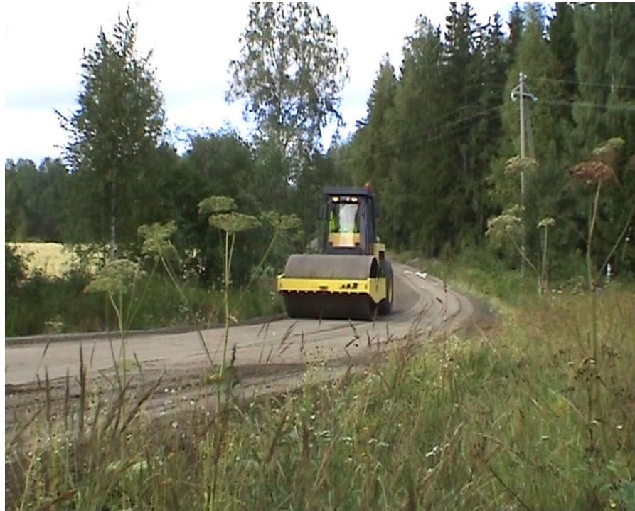
Figure 10: Fibre-ash course is being compacted with a roller
