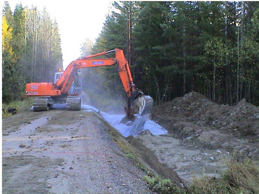
Figure 13: After removing of the soil the fibreclay is being spread to construct the hydraulic barrier
