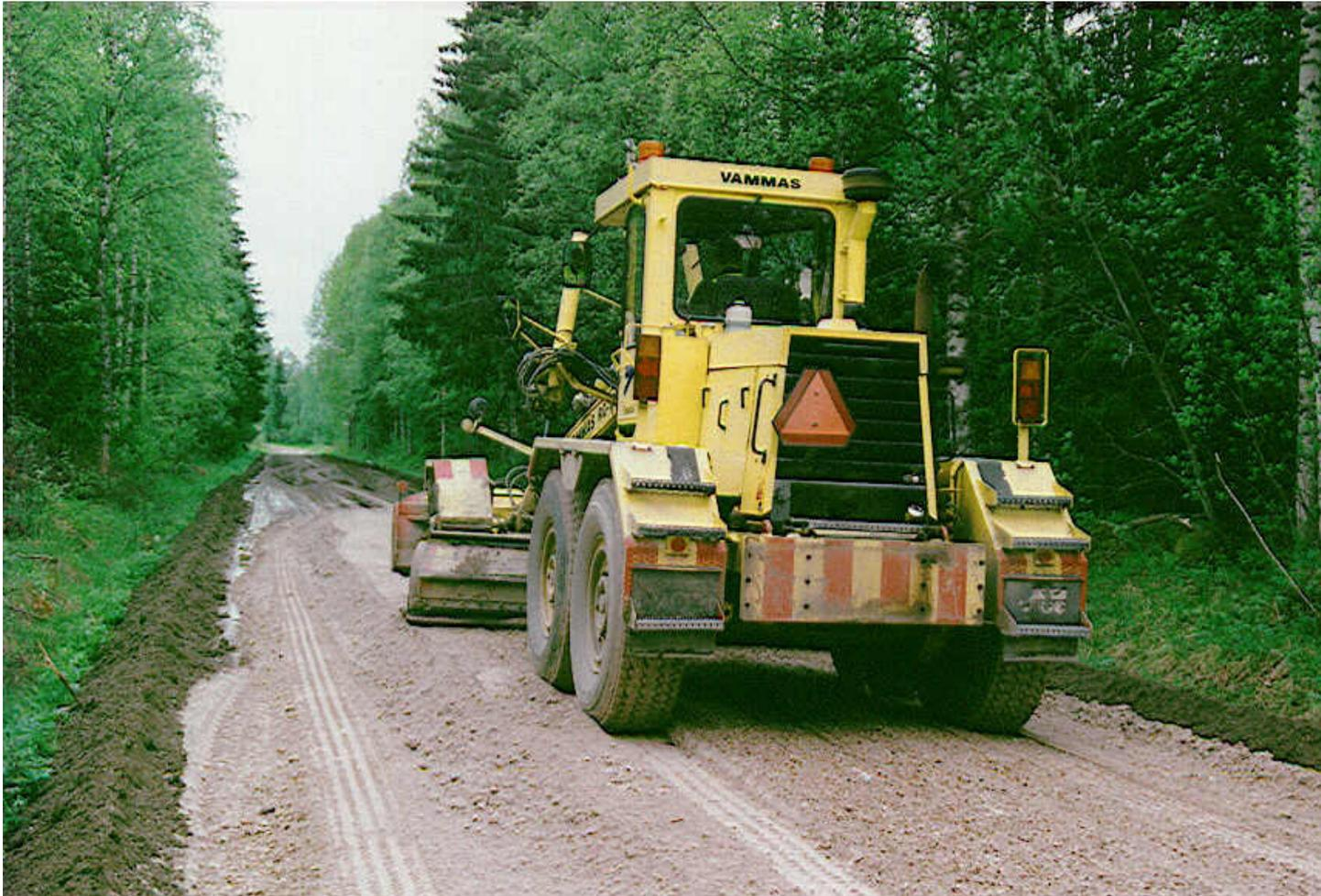
Figure 6: Covering course with filtercake-stabilised crushed stone
