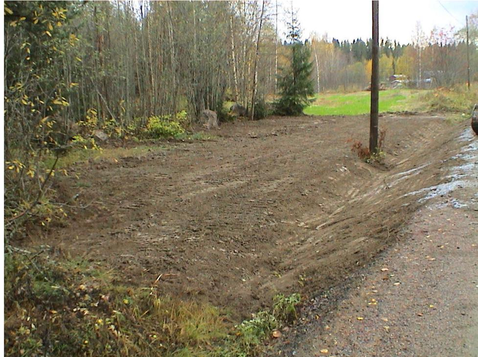
Figure 14: The hydraulic barrier course is covered with the original soil material from the site
