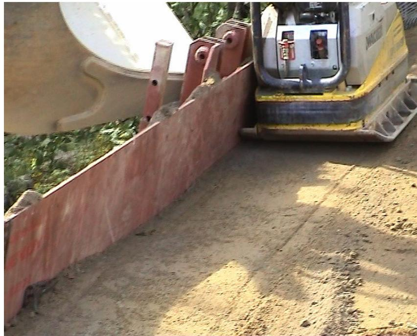
Figure 23: The fibre-ash course is covered thinly with crushed aggregate, and the safety lane can be compacted
