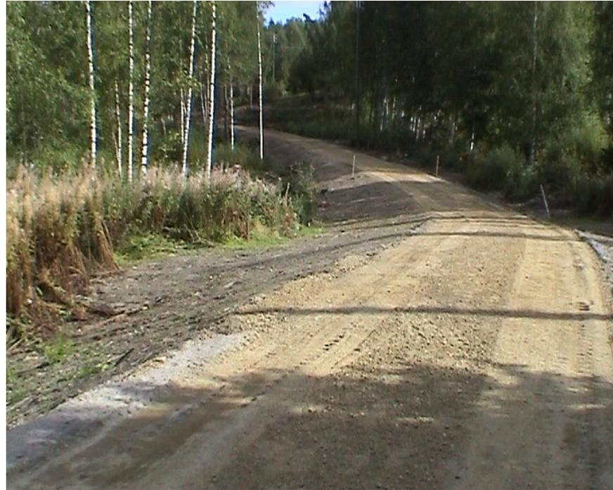
Figure 18: The light-traffic lane (and the fibre-ash course)
